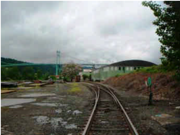
View from the Eastern Portion of the Site
