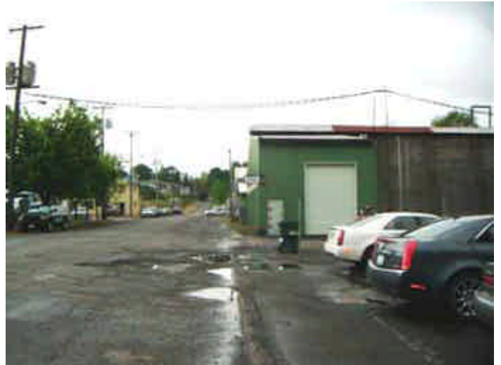
Exterior Warehouse View
